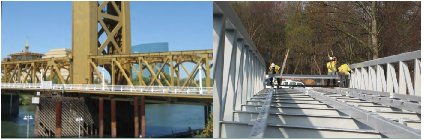
Figure 30— Example of a Solway Bridge solution using FRP deck construction. Left example is Tower Bridge in Sacramento. Image courtesy of Composite Advantage
