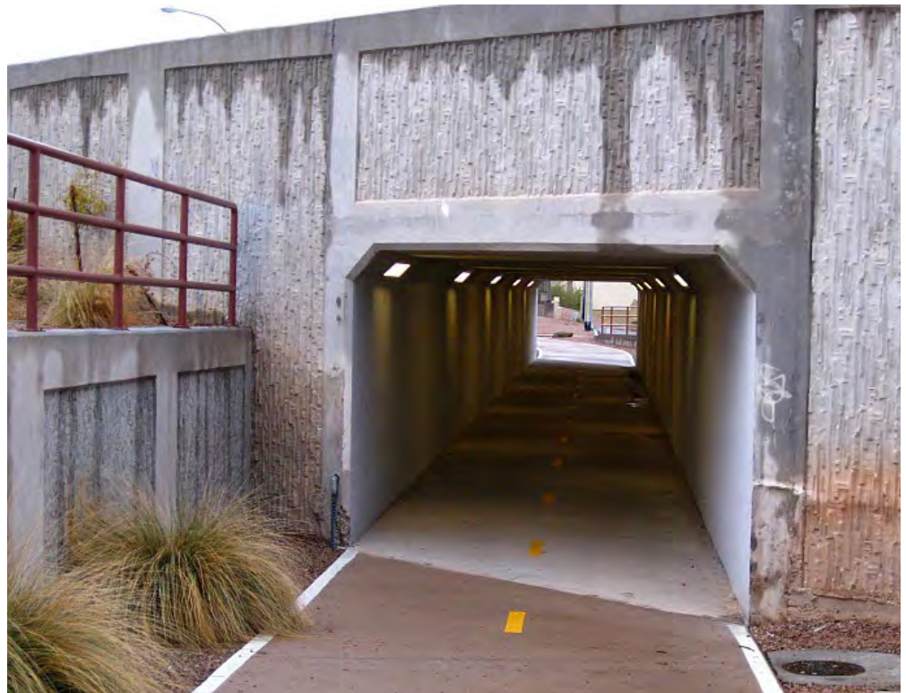
Figure 9—Example of a below-grade greenway underpass (“cut and cover”) that can be utilized to cross under Lovell Road.
