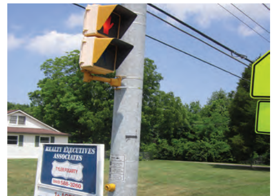
ADA-compliant signal upgrades at the intersection of Cedar Bluff Road and Fox Lonas Drive would include countdown signal heads and accessible pushbuttons.
